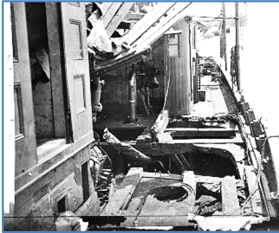
Damage due to boiler explosion
